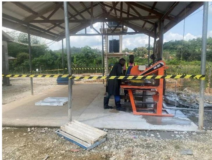
Figure 10.15 – Core Cutting Area
